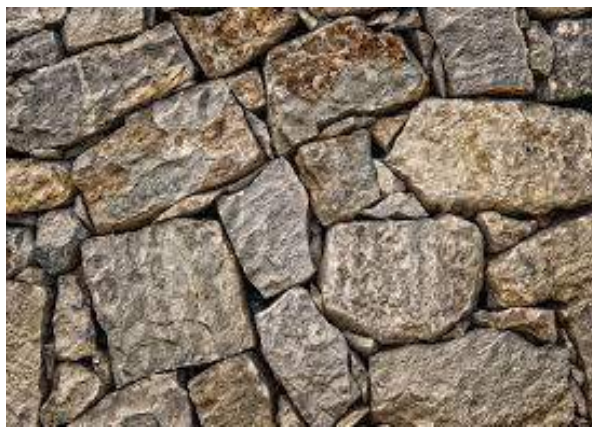
Fig3. Stone masonry wall
