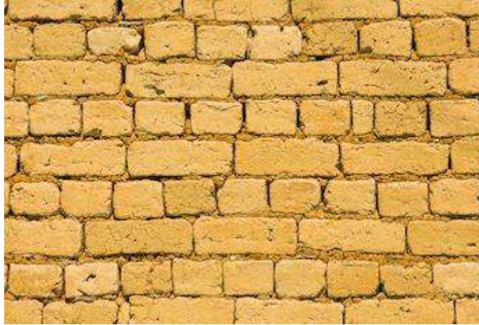
Fig. 6: Brick work in mud
